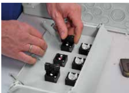
Install and wire built-in devices.
