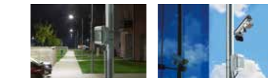
Lighting control of a residential complex and parking
